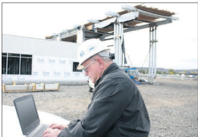
Dan Lewis, an electrical inspector with Crook County. Opinions by the Oregon Department of Justice and Legislative Counsel indicate many small cities may have to either shut down building programs or hire building officials with three-digit salaries.
