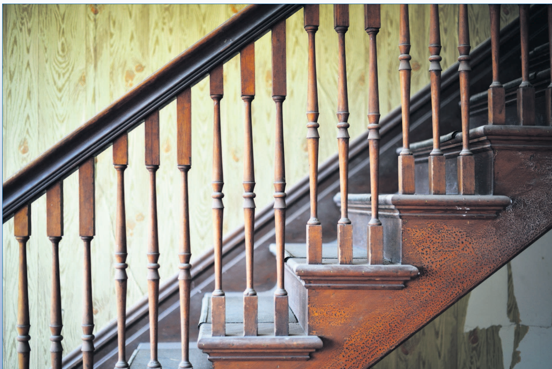
The original railing on the staircase in the grand room of the 120-year-old Victorian house being renovated in Pendleton. The house was moved from the Pendleton County Club in 1996. Staff photo by E.J. Harris
