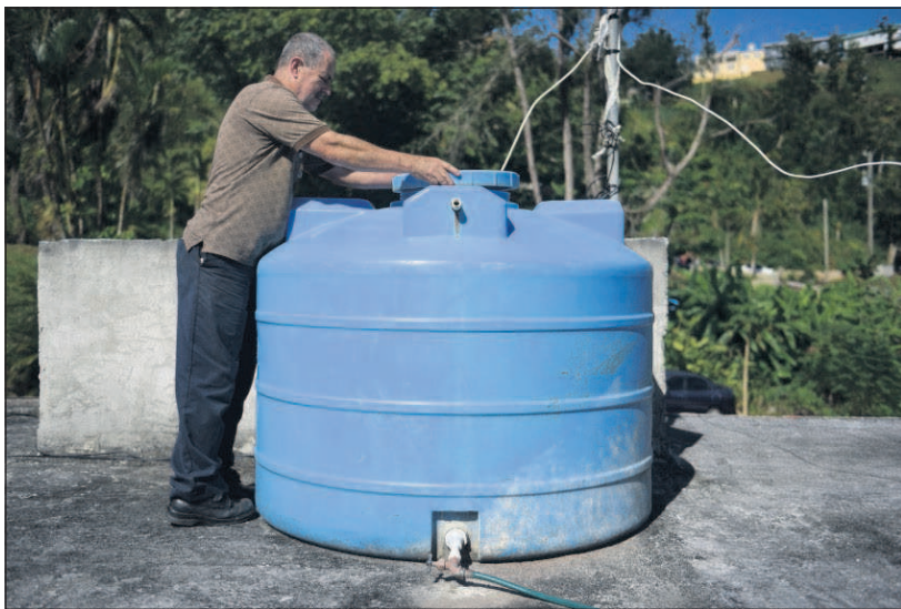
José Morales checks a water tank installed on the roof of his residence in the Barrio Mana neighborhood, in Corozal, Puerto Rico. After Hurricane Maria shredded the electric poles in this plantain farming town, Barrio Mana residents asked federal officials but never received a generator to pump water from the well that supplies more than 100 families.
