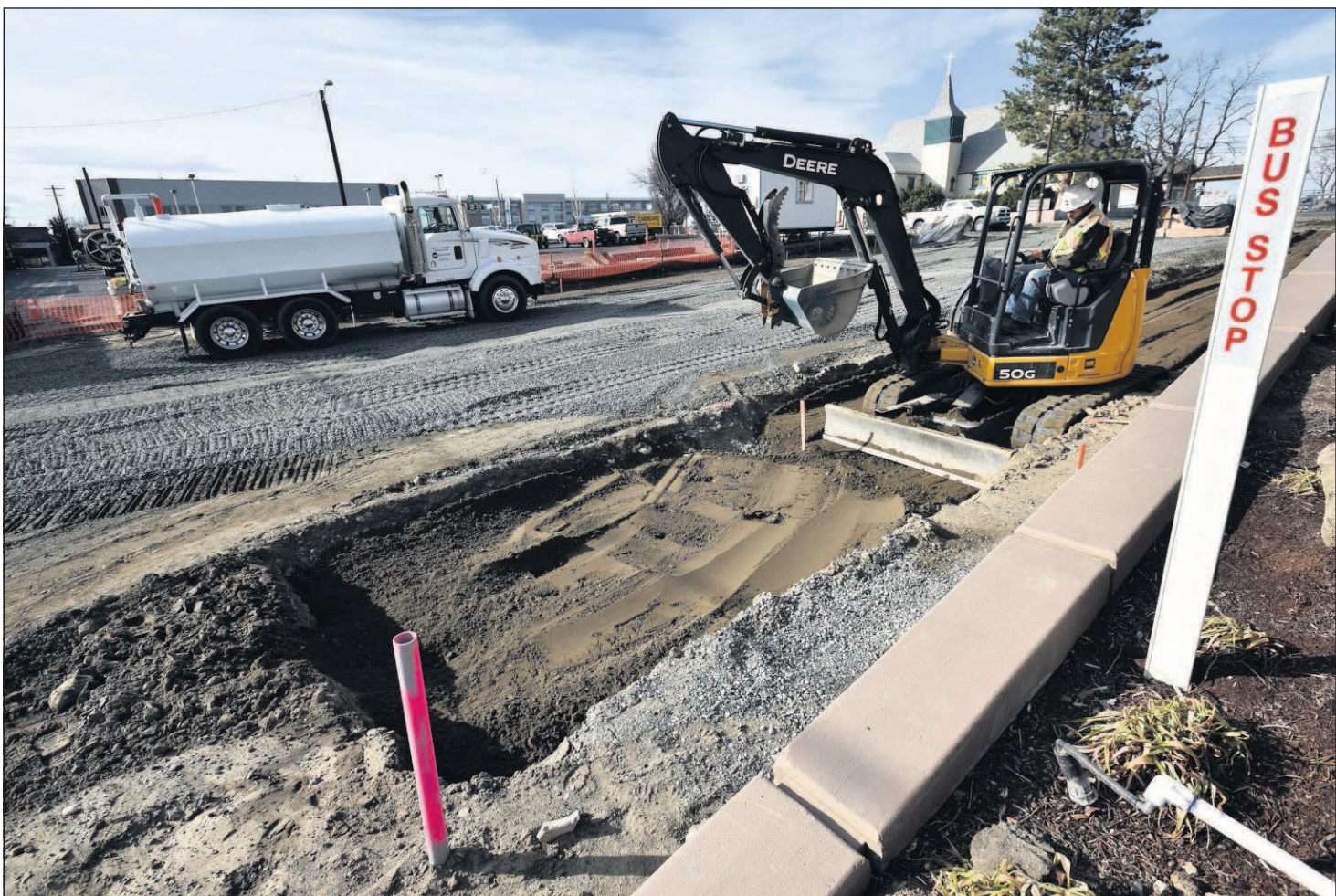
A small excavator levels dirt while working on the festival street site Tuesday in Hermiston.
