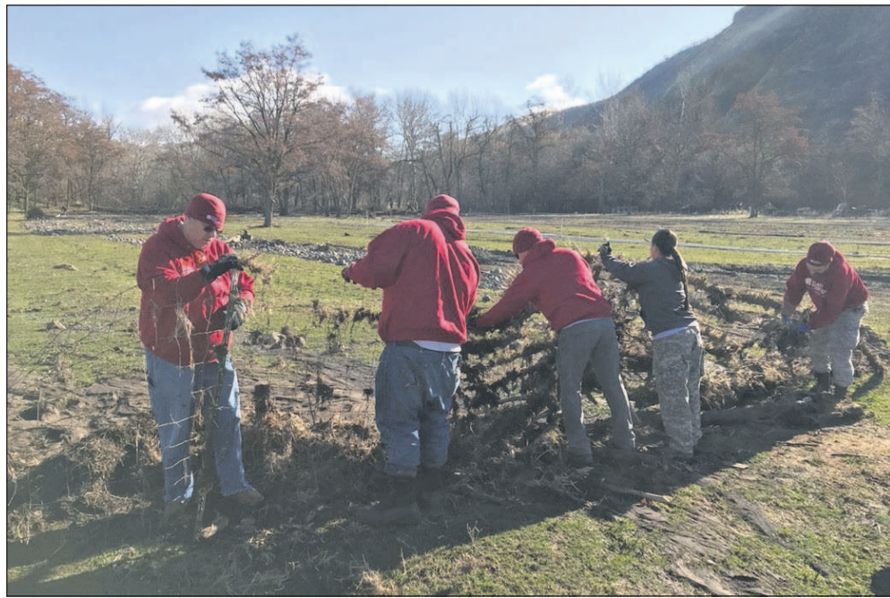
Photo contributed by Umatilla County Emergency Management Volunteers and members of the nonprofit disaster relief organization Team Rubicon work Saturday to clear fencing from flood debris on a home near Milton-Freewater.
