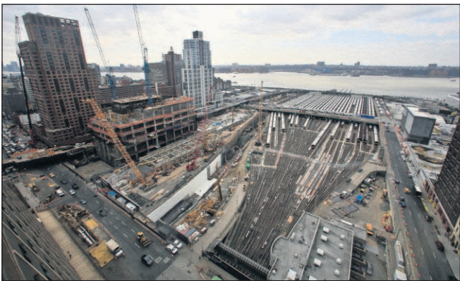
This 2014 file photo of the Hudson Yards project site shows ongoing construction of a rail tunnel, center left, at the Hudson Yards redevelopment site in New York.
