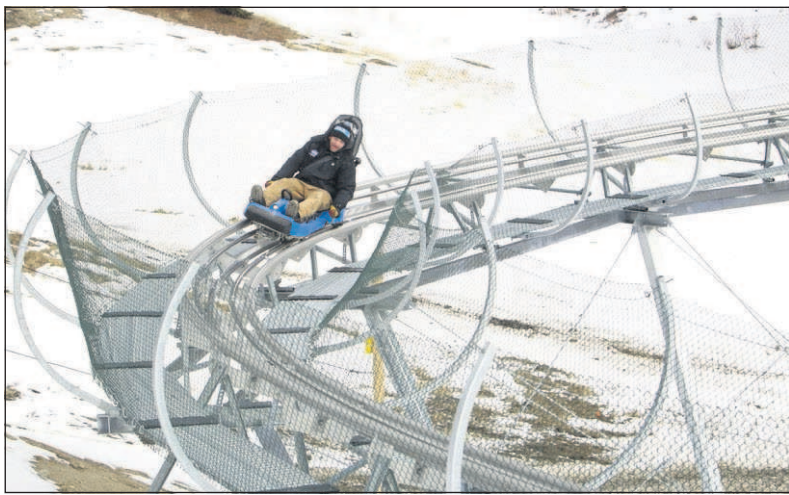
The Glade Runner mountain coaster at Bogus Basin has a top speed of 25 mph. It's gravity run, and each sled has brakes operated by the rider.
