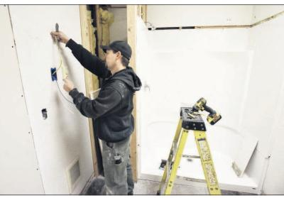
Staff photo by E.J. Harris Jon Dickerson with Pendleton Electric installs wiring for a fan in a shower room at the Pendleton Warming Station.
