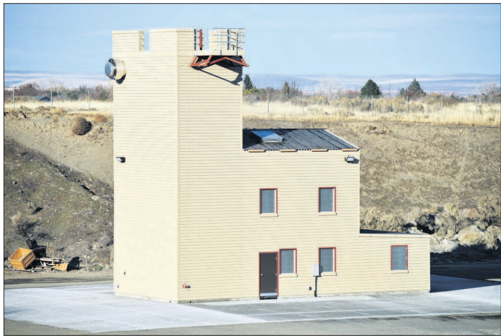
Construction is complete on a new training tower at the Umatilla County Fire District 1 substation off of Westland Road outside of Hermiston. Staff photo by E.J. Harris
