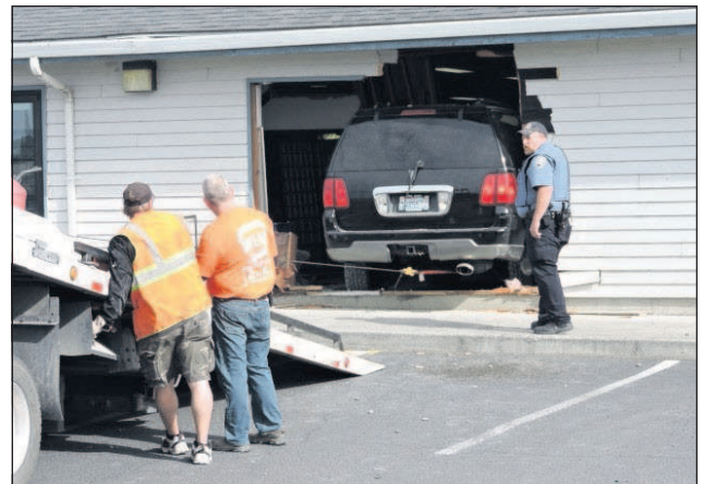
Staff photo by Jade McDowell A black SUV is towed from inside the Umatilla Post Office after it crashed through the side of the building Saturday just before noon, destroying mailboxes and parts of the building.
