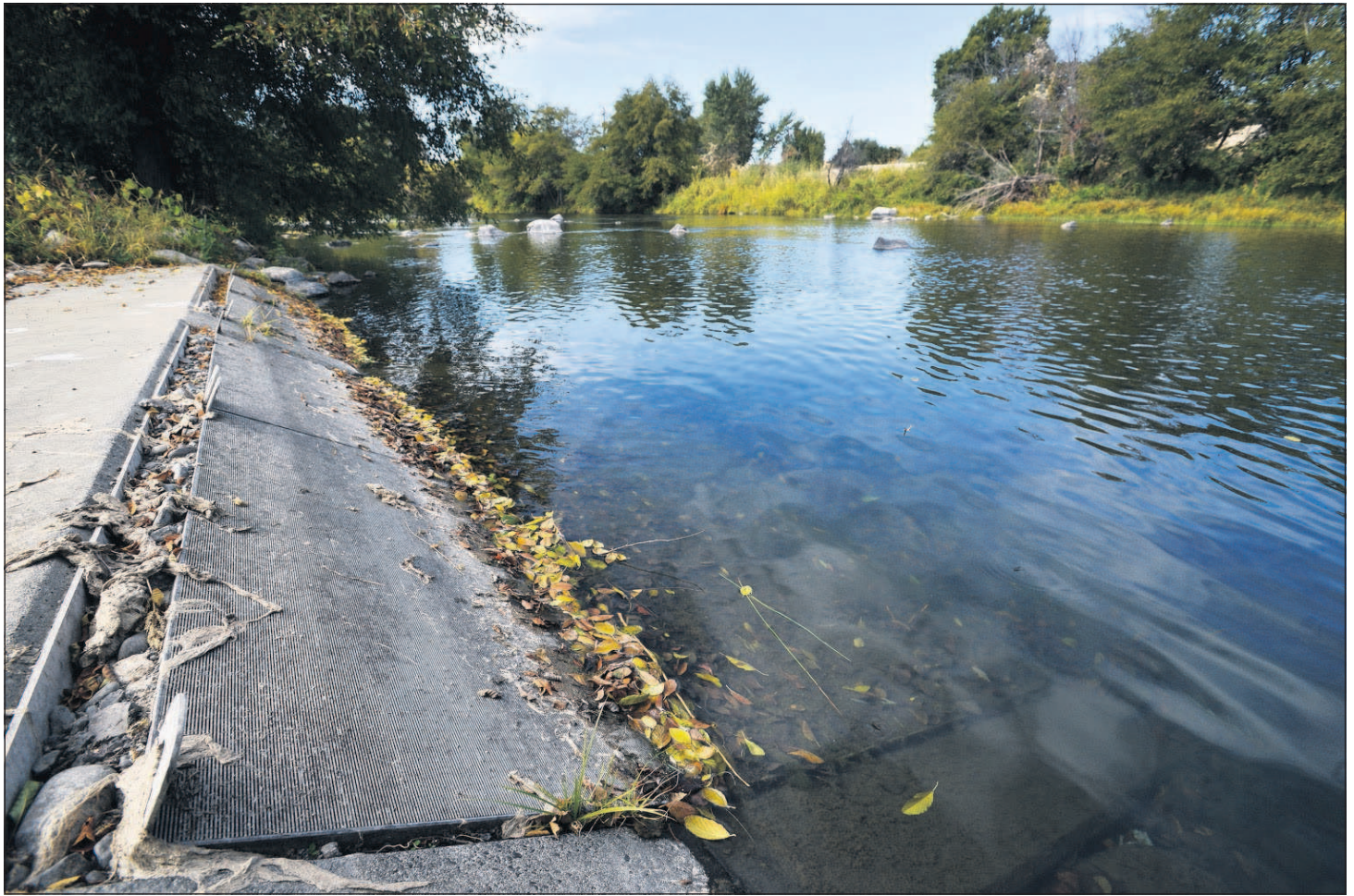
The intake for the city of Pendleton's aquifer recharge system takes water from the Umatilla River east of Pendleton during the higher rates of flow. Staff photo by E.J. Harris
