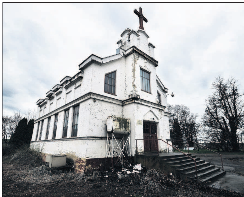
Constructed in 1913 in the Portuguese Colonial Revival style, the old St. Peter's Catholic Church in Echo has sat empty for 20 years. The Fort Henrietta Foundation and Echo Kiwanis are hosting an open house Sunday from 2-4 p.m.
