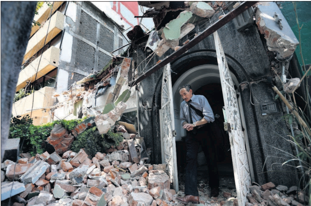
AP Photo/Marco Ugarte A man walks out of the door frame of a building that collapsed after an earthquake in the Condesa neighborhood of Mexico City on Tuesday.
