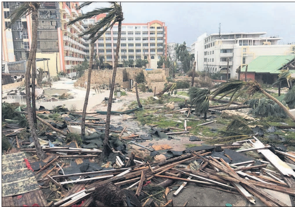
This Sept. 6 photo shows storm damage in the aftermath of Hurricane Irma on the Caribbean island of St. Martin.
