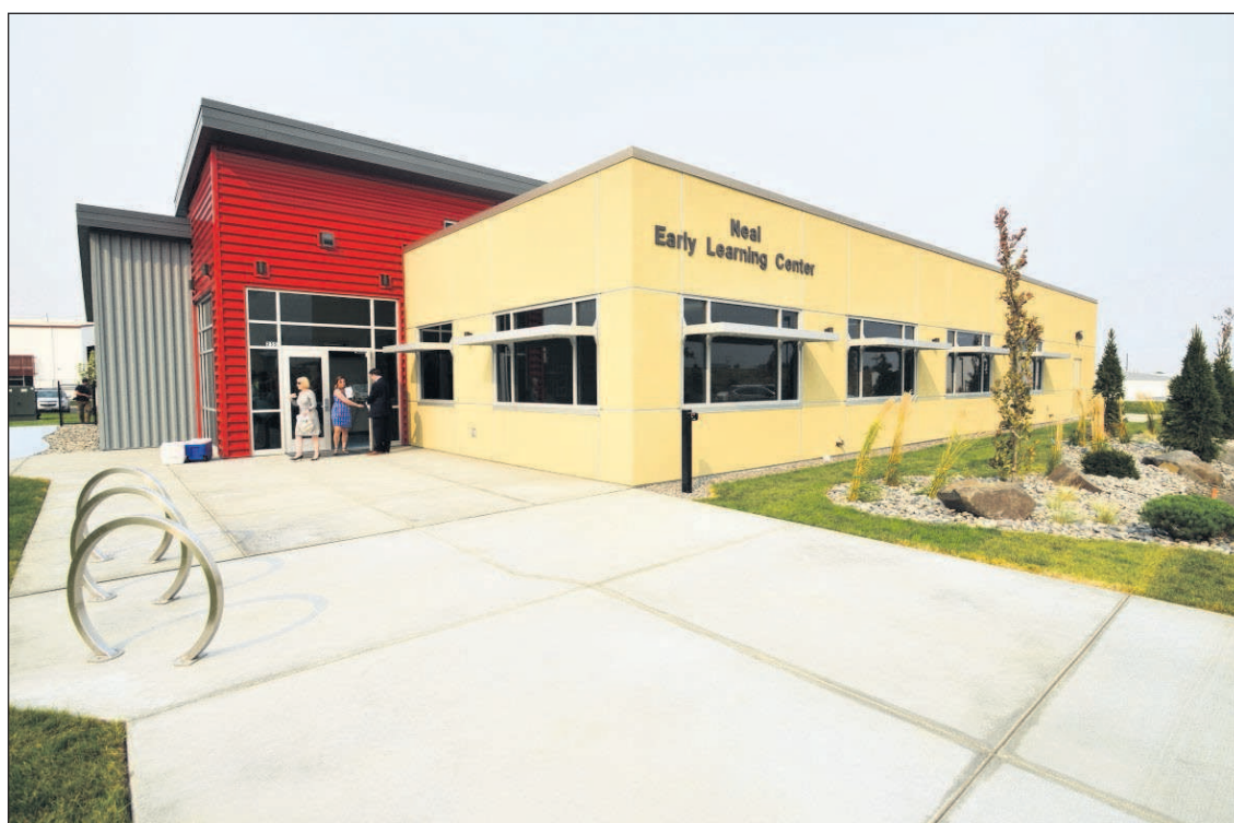
The Neal Early Learning Center is a collaborative effort between the Port of Morrow, InterMountain Education Service District, the Morrow County School District and Umatilla-Morrow Head Start.
