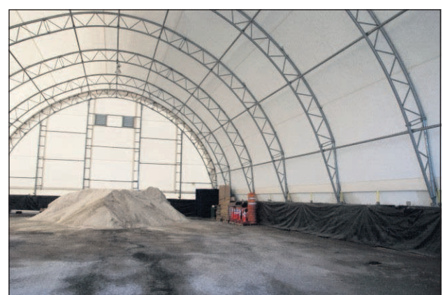
Contributed photo by ODOT This salt shed in Jordan Valley is being replicated by ODOT at eastern Oregon locations, including Pendleton and Irrigon.
