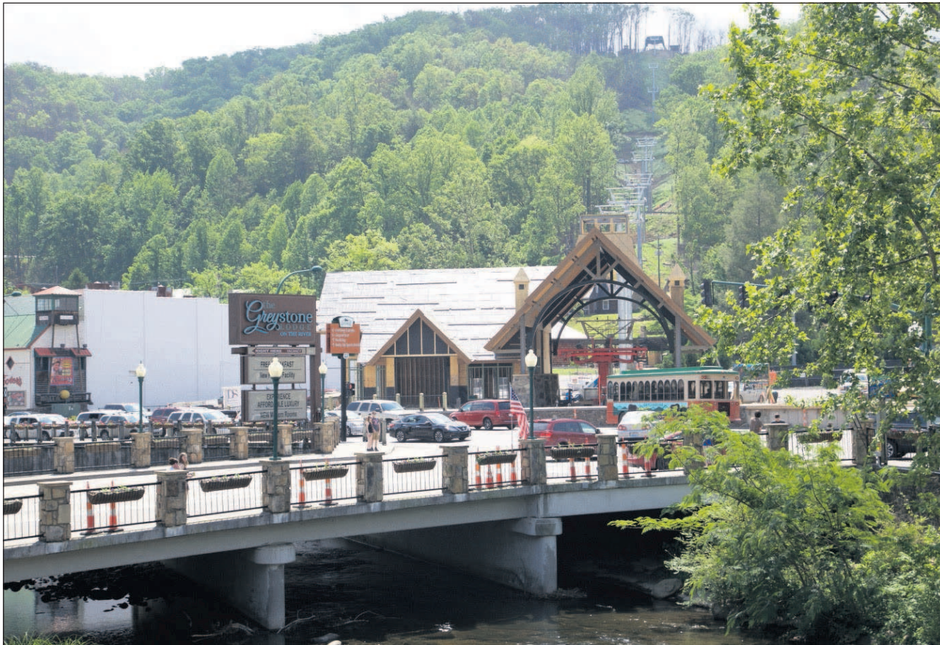
In this May 20 photo, a new chairlift attraction is under construction in downtown Gatlinburg, Tenn. A deadly wildfire in November 2016 put a dent in the tourism industry there, but signs of growth are returning.
