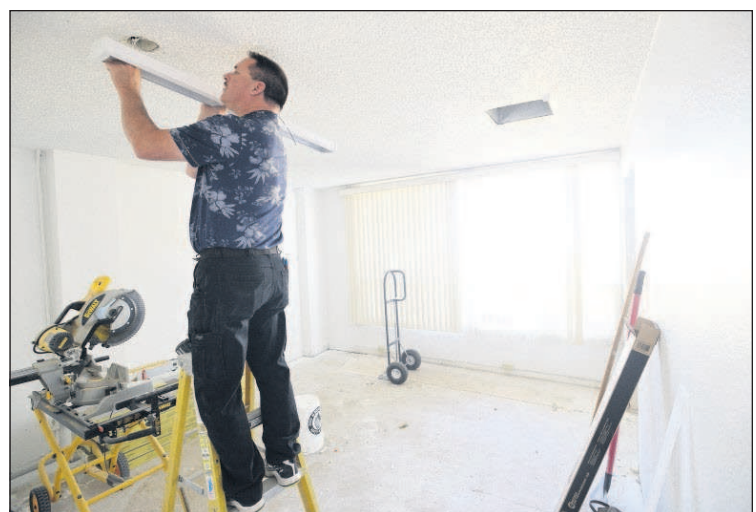
Umatilla County maintenance supervisor Mark Tanner installs a new light fixture in the county office Wednesday in Milton-Freewater.
