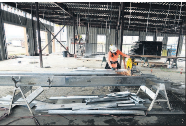
Staff photo by E.J. Harris Dion Fry, with All Wall out of Post Falls, Idaho, cuts framing for a wall while working on the new Yellowhawk Tribal Health Center on Friday in Mission.
