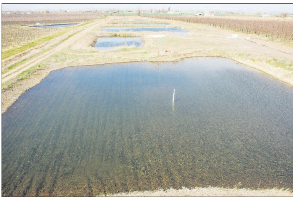
Photo contributed by the Walla Walla Basin Watershed Council The Johnson Aquifer Recharge Site near Milton-Freewater is roughly three acres in size, and has been in operation since 2004.
