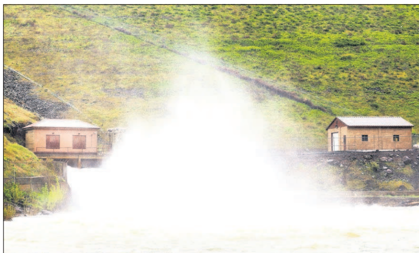
Staff photo by Kathy Aney Water pours through a spillway on the backside of McKay Dam on Wednesday at a rate of 1,160 cubic feet per second. The Bureau of Reclamation may start tapering off by Friday.
