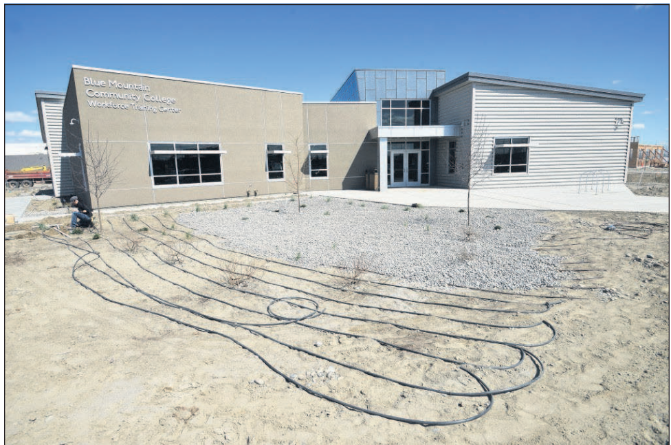
The finishing touches are still being applied to BMCC's new Workforce Training Center as classes begin Monday in Boardman.
