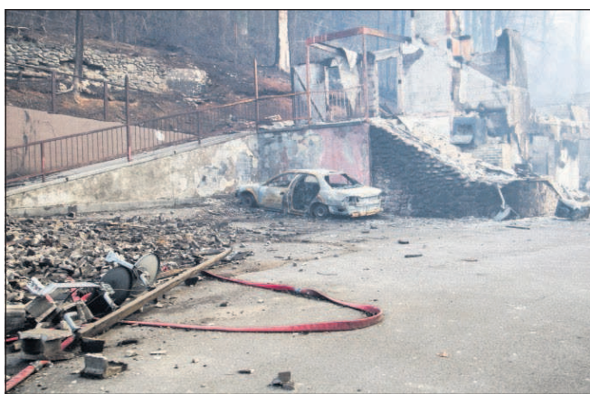
A scorched vehicle sits next to a burned out building in Gatlinburg, Tenn., on Tuesday.
