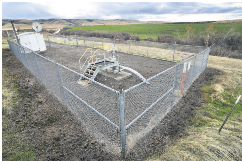
A value station for the Tesoro Logistics petroleum pipeline stands in a field off Cayuse Road east of Pendleton.
