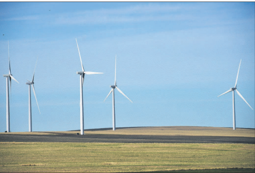
The 10-megawatt Chopin Wind Farm is up and running north of Weston.
