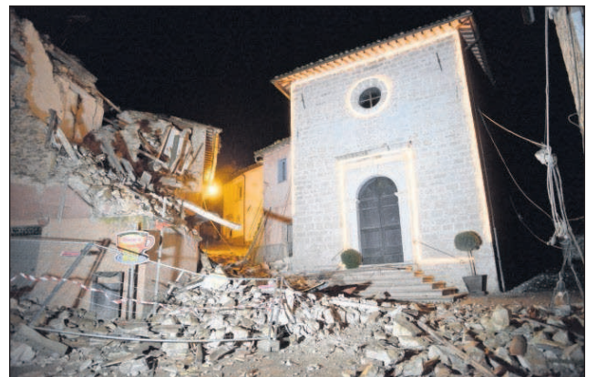
The Church of San Sebastiano stands amidst damaged houses in Castelsantangelo sul Nera, Italy, Wednesday following an earthquake.
