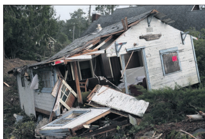
Debris is strewn about after a tornado struck Manzanita on Friday. Dave Killen/The Oregonian via AP
