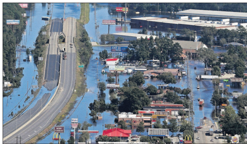
Floodwaters from Hurricane Matthew covers parts of Interstate 95 and homes and businesses in Lumberton, N.C., Wednesday.
