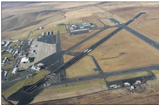
This November 2008 file photo shows the Eastern Oregon Regional Airport in Pendleton.
