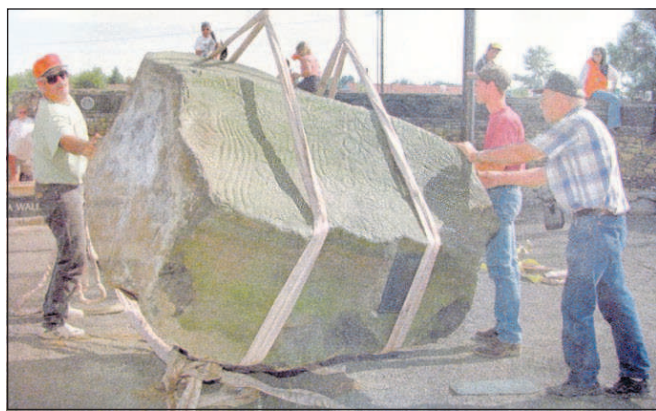
In this July 1996 EO file photo, Ken White, left, of the maintenance department of the Confederated Tribes of the Umatilla Indian Reservation, works with Kai Bolen, center, and Leon Shockman, both of Shockman Brothers crane contractors, to place the 10-ton Wallula Stone in the center of the Niix-Ya-Wii Veteran's Memorial in Mission.
