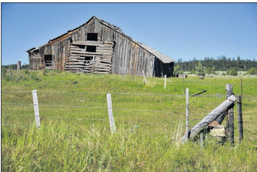
19 Mile 267.8 - An old barn south of Fox.
