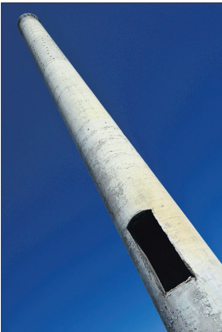
10 Mile 152.2 - A smokestack at a demolished mill in Hines on Highway 395.
