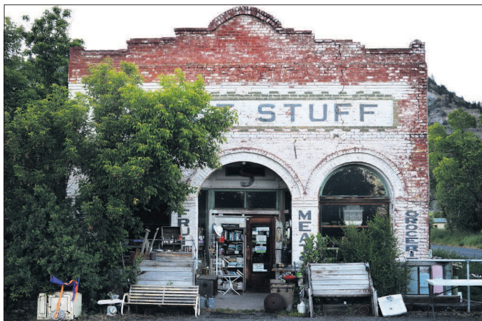
1 Mile 0.0 - An old brick store in New Pine Creek at the Oregon-California border on Highway 395.
