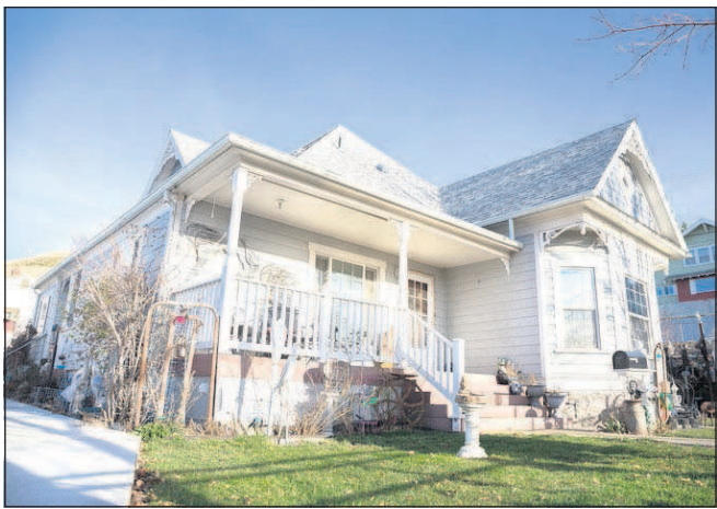
Staff photo by Kathy Aney The owners of this house on Southeast Third Street are suing the city of Pendleton for $200,000 as compensation for flood damage sustained from a leaky water line on Nov. 28, 2013.
