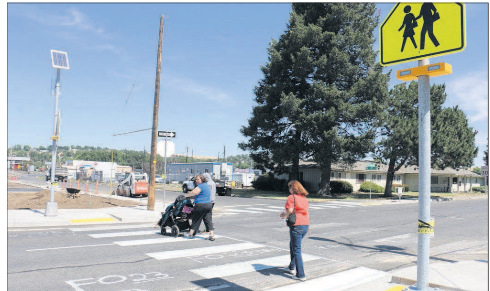
Frazer Ave., Pendleton pedestrian upgrades include rapid flash crosswalk beacons.
