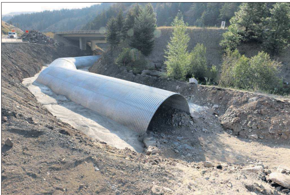
Ladd Creek culvert prior to construction of freeway undercrossing.
