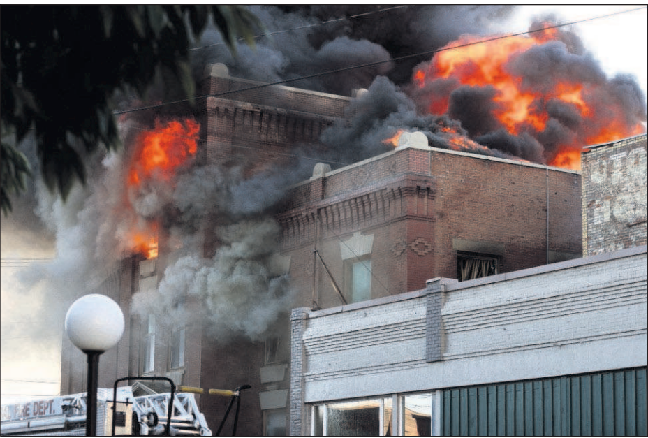
3 Flames erupted from the roof of the old City Hall building in July in Pendleton. Staff photo by E.J. Harris
