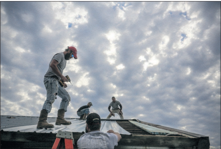
Stephen B. Thornton/Arkansas Democrat-Gazette via AP Construction workers John Croft, left, Michael Edwards, top center, Lee Croft, top right, and Jacob Croft, bottom center, repair damage to the roof of a chicken house, Wednesday along Arkansas 247 north of Atkins, Ark.
