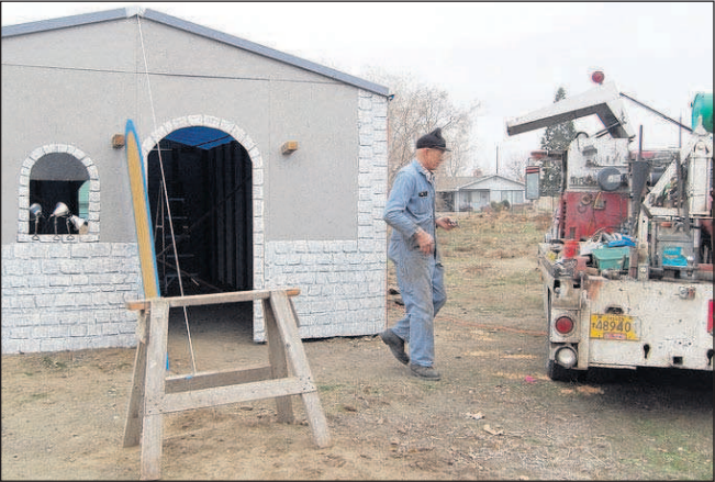
Staff photo by Tammy Malgesini Larry Hanson works by a newly constructed building that will house Gamaliel for this weekend’s Journey to Bethlehem at the Hermiston Seventh-day Adventist Church.
