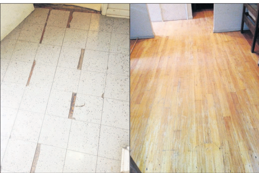
Photos contributed by Michele Madril Tile flooring containing asbestos (left) was recently removed to reveal the original Douglas fir wood floor (right) at Corporation Bunkhouse, which houses female students for Pendleton Outdoor School on the Umatilla National Forest.
