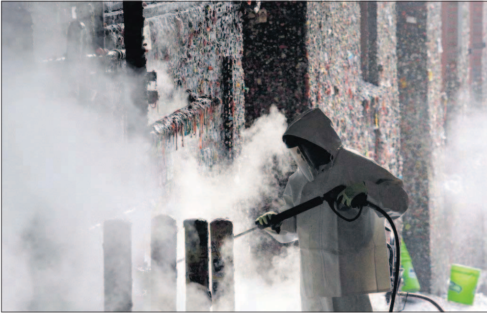
A worker uses a powerful steam cleaner to work decades of gum off a "gum wall" that stretches behind and above him, Tuesday in Seattle. Tourists and locals have been sticking their used chewing gum to the wall near Pike Place Market for 20 years, leaving an estimated 1 million pieces in a kaleidoscope of colors, some stretched and pinched into messages, hearts and other designs.
