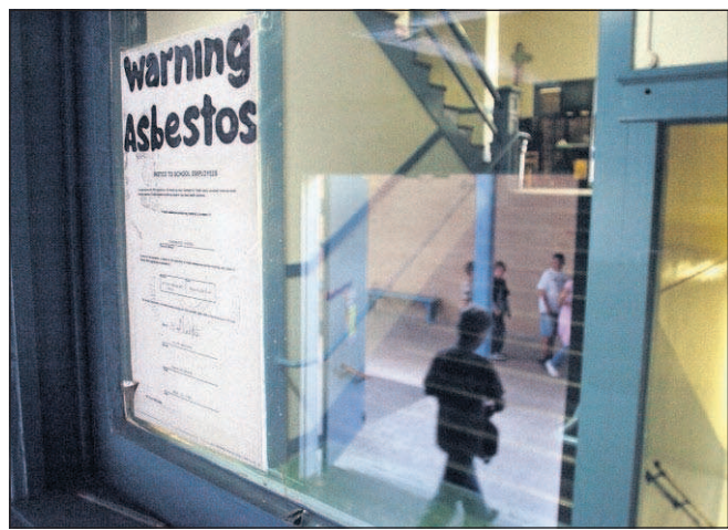
A warning for asbestos is taped on the door of Freewater Elementary in Milton-Freewater in this May 2007 file photo. The Milton-Freewater School District has received a $15 million grant to build a new school, contingent on raising at least $12.5 million of its own.
