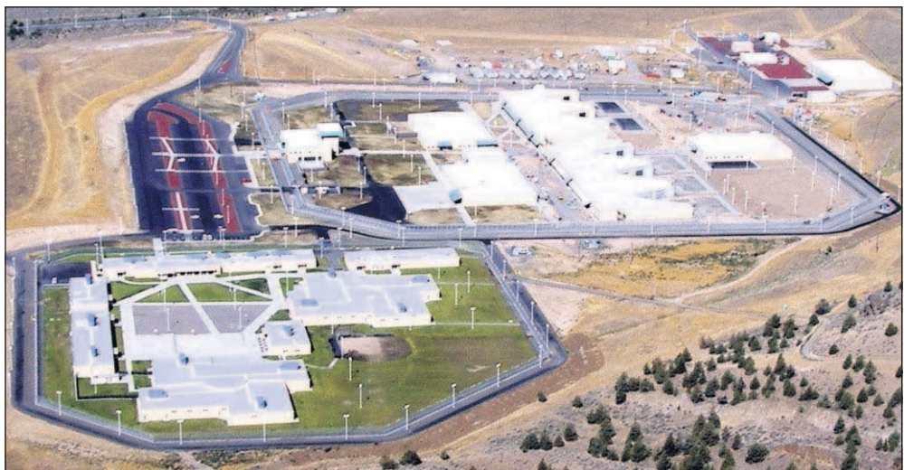
The Deer Creek Correctional Institution in Madras. DOC wants to renovate the facility to accommodate an increase in inmate population. The $9.5 million needed to expand and staff the facility would come from a program designed to keep parolees out of prison.
