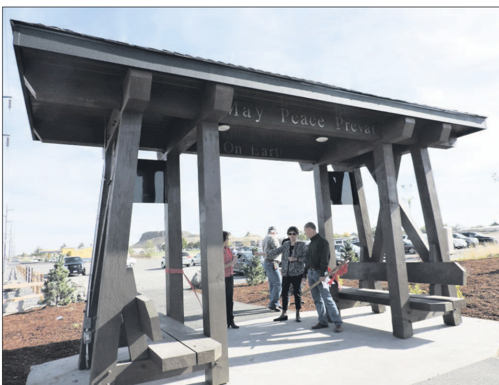
A new arch towers over the entrance of Oxbow Trail. A drinking fountain will be added in the spring.
