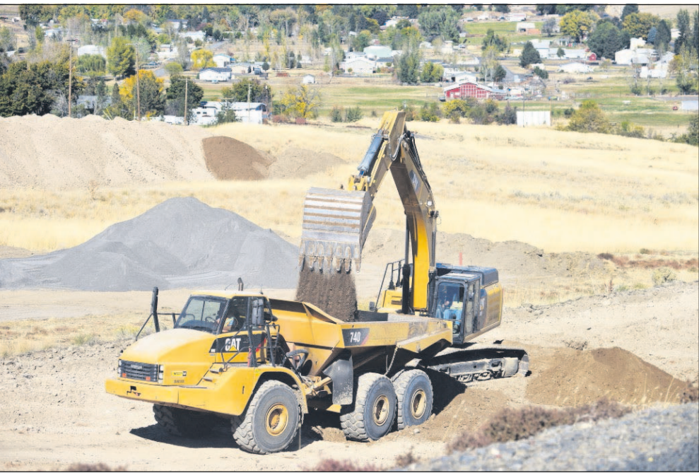
Staff photo by E.J. Harris An excavator drops a load of dirt into a dump truck near the top of the McKay Reservoir Dam on Tuesday in Pendleton. The Bureau of Reclamation is replacing a toe drain that collects water seepage from the dam and redirects the water into McKay Creek.
