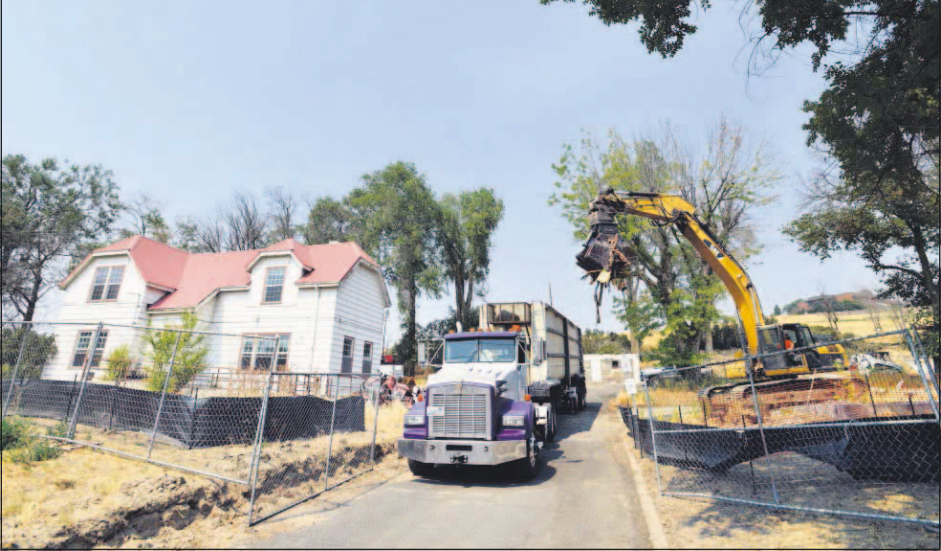
Staff photo by E.J. Harris An excavator with 3 Kings Environmental Excavations out of Battle Ground, Wash., removes debris while demolishing one of the structures at Pendleton Cottage on Monday in Pendleton.
