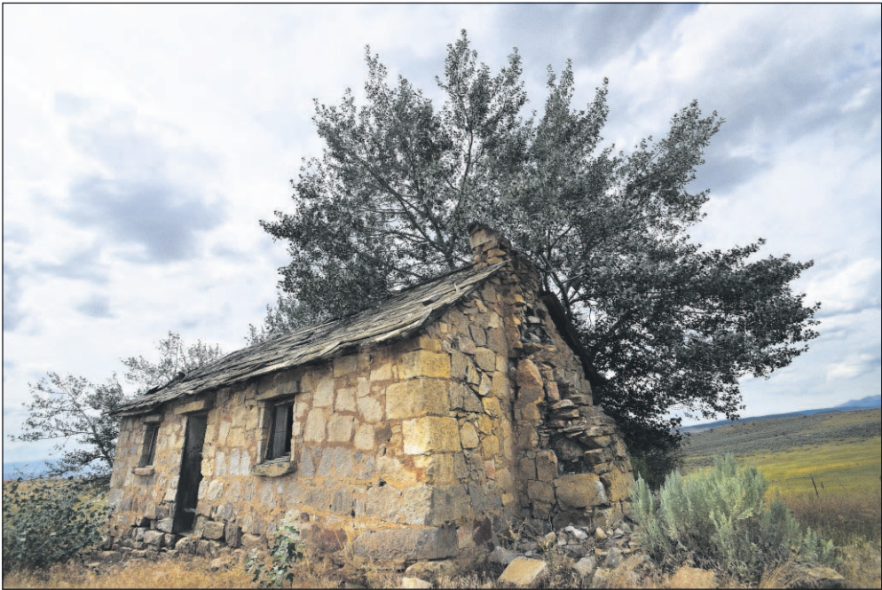
A solitary one-room homestead build of volcanic tuff stands off Sparta Lane just outside of the town of Sparta.
