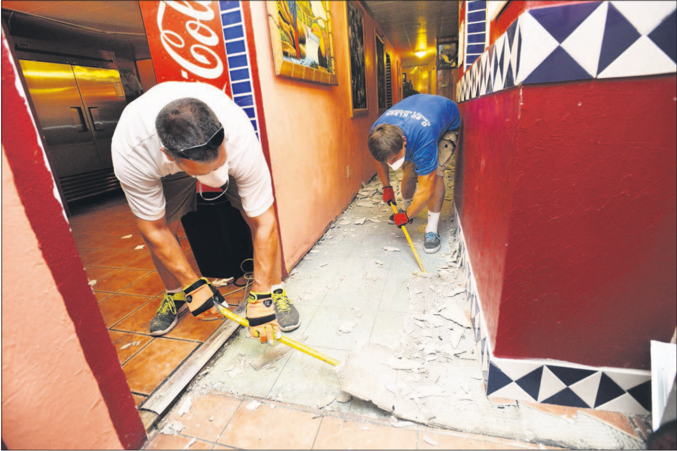
Rob Markwick and C.J. Flores, with O So Kleen of Hermiston, tear out water-damaged floor tiles with crowbars on Tuesday at Joe's Fiesta on Main Street in Pendleton.
