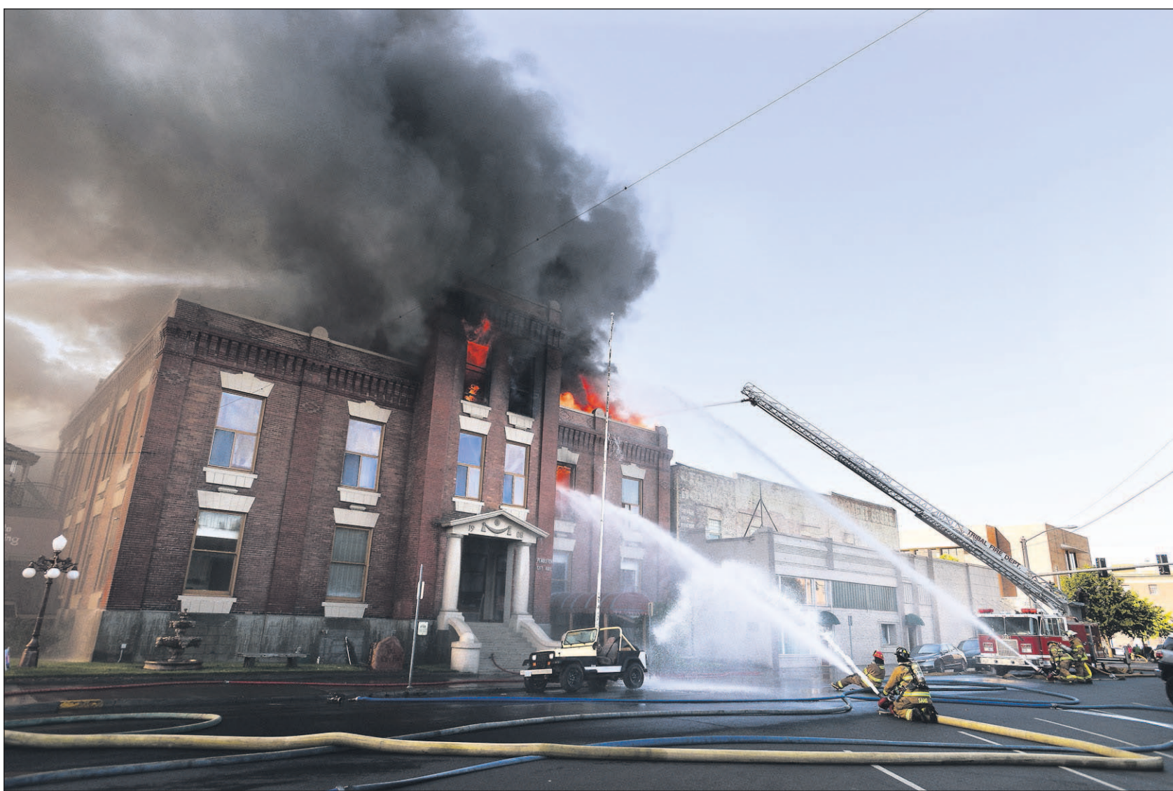
The old city hall building burns on the corner of southeast First Street and Dorion Avenue as firefighters from all over Umatilla County battle the blaze Tuesday in Pendleton. Staff photos by E.J. Harris
