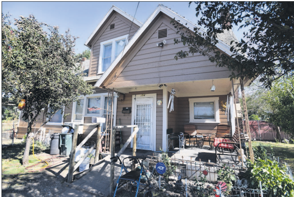
The home of Dorothy and Leonard Bullock has a fresh new coat of paint on Monday after volunteers came together and gave the house a fresh coat.
