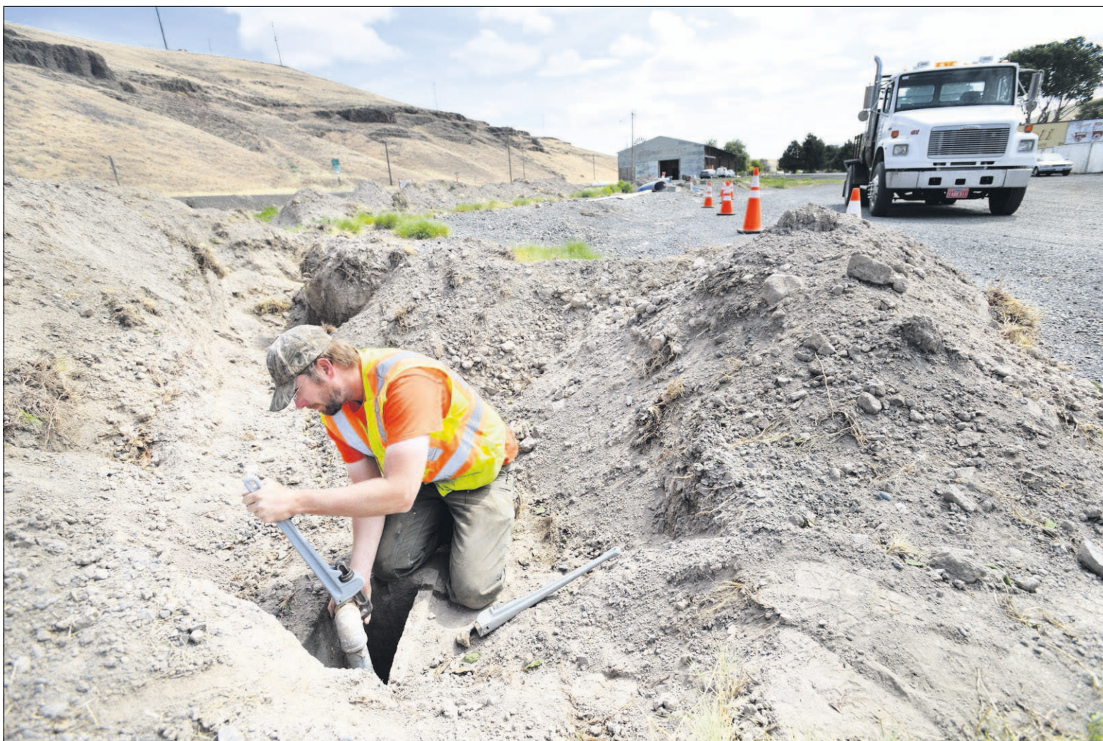
Ione maintenance supervisor Curtis Thompson uses a wrench to tighten a new coupling to a waterline while installing a new stand-pipe Wednesday at the Morrow County Grain Growers store in Ione.
